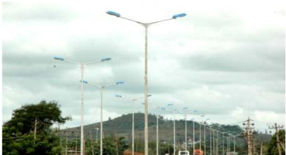
Photo 2 : 120W Induction Lamp Street Lights in Gadag City - in Replacement of 250W HPSV.
