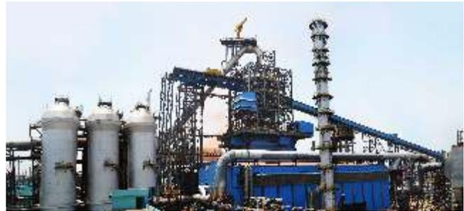
Coal Dust Injection (CDI) system was operationalized in Blast Furnace-4 of Rourkela Steel Plant recently. This latest operational facility will result in improvement of techno economic parameters and enhance productivity of hot metal in the Blast Furnace.
