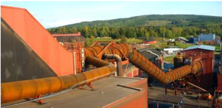
Sweden-based Uddeholm AB Hagfors, manufacturer of tool steel for industrial tools, has successfully commissioned phase one of the modernisation of the EAF fume treatment plant with latest filter technology from SMS group. As phase one of the project, SMS group upgraded the roof canopy installing a high-efficiency EAF fume evacuation hood – the patented SMS Frustum, replaced the existing secondary duct system, installed a highly efficient axial cyclone and a new pulse jet filter.
