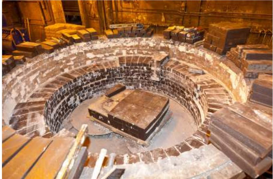
needs to be made stronger. In that respect a binder containing calcium magnesium aluminate has proven to be more resistant to penetration and corrosion. Calcium magnesium aluminate is a new generation of binder that provides highly reactive spinel and develop unique micro structure and gives rise to superior corrosion resistance. This binder at the same time displays a unique placing property and make the castable a robust one.
