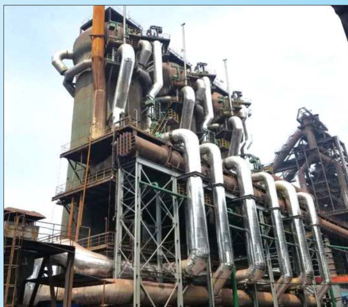
Internal combustion chamber stoves for 1497m 3 BF at JianLong Steel converted into Yuxing top fired with a catenary dome
