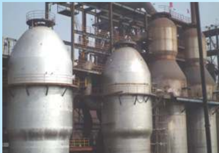
Conventional 3-section top fired transformed into Yuxing top fired with a catenary dome by cutting the top portion of the existing stove shell
