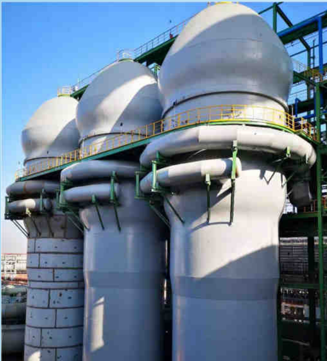
Yuxing top fired stoves with a catenary dome for 2x2850m 3 Bfs
