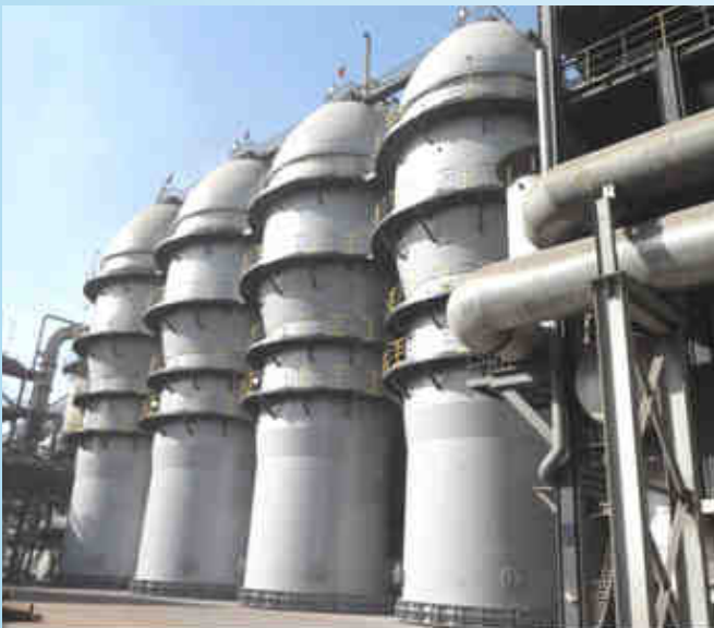
Yuxing top fired stove with a catenary dome achieved monthly mean HBT of 1314.7 oC
